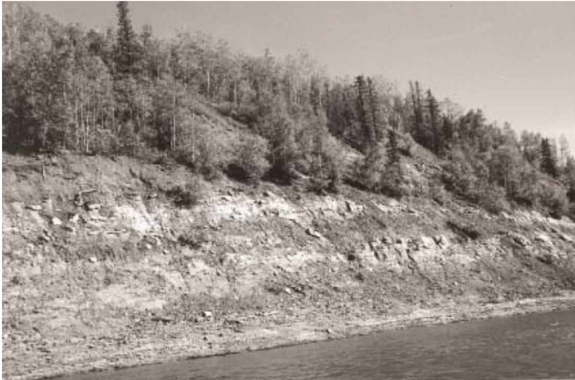
Figure 9.12.4a. Overview of slumped Sinkhole South Section, Athabasca River.
