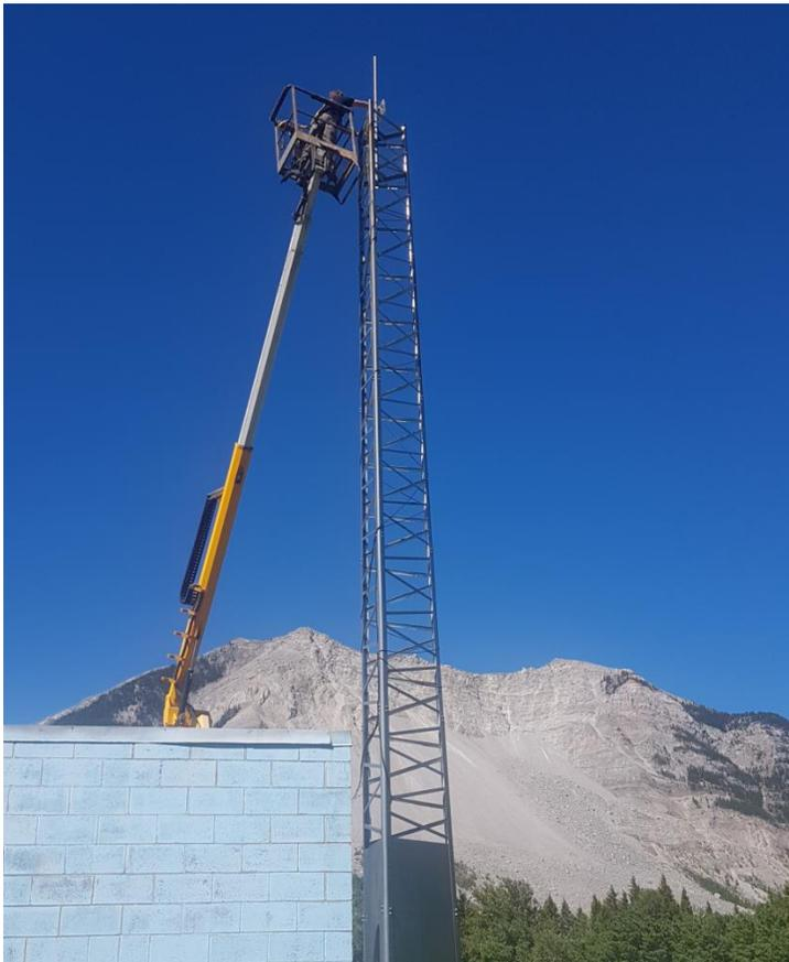
Figure 4. Testing the RSSI value from the top of the pump house antennae towards the FSIC.
