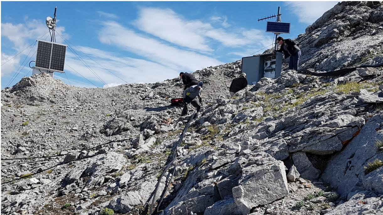
**Figure 5. AGS field crew dismantling the borehole hub and conduit lines leading to multiple monitoring equipment locations.**
