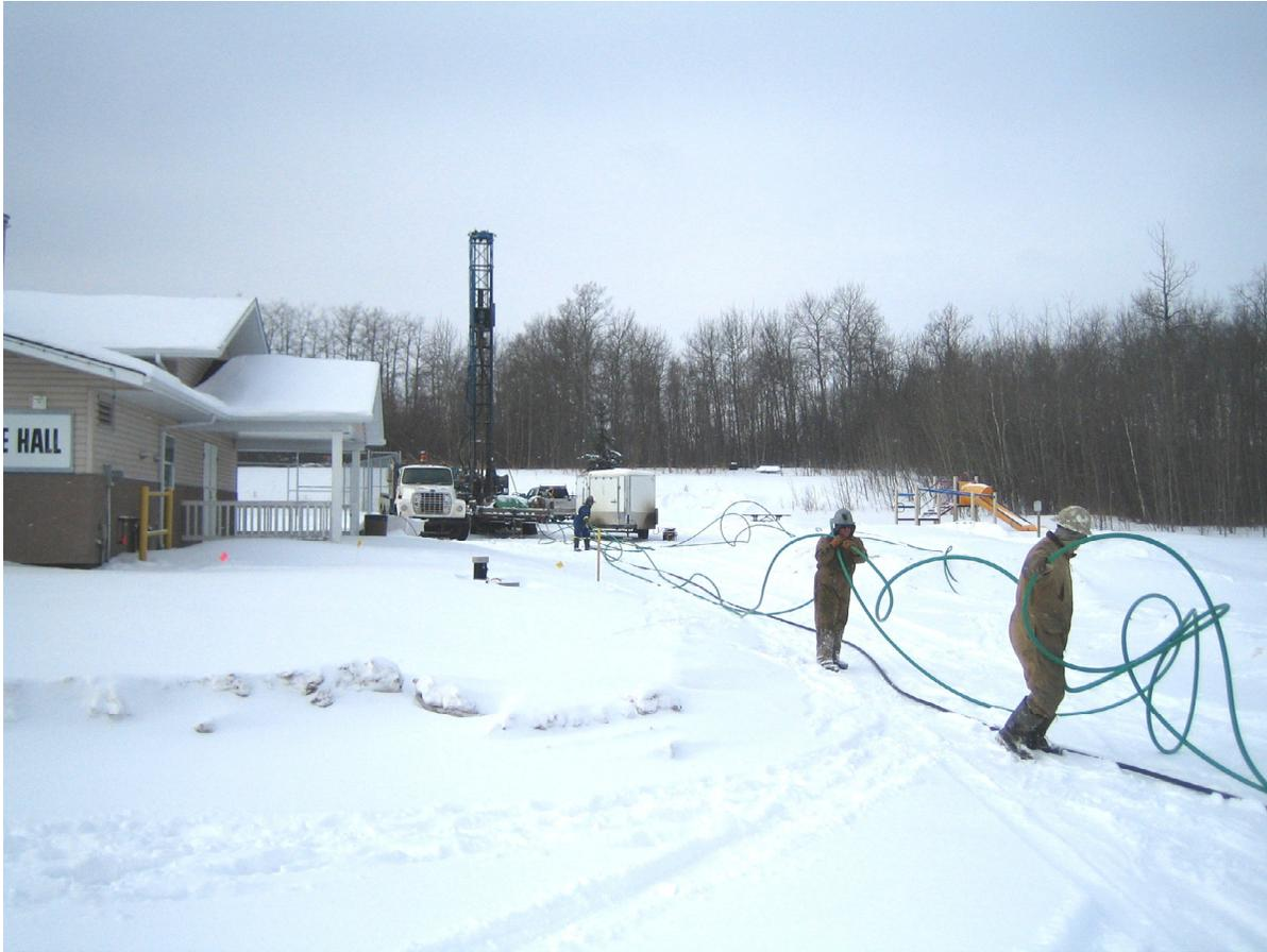
**Figure 5. Hastings Lake Community Hall with drill rig in background and u-bend heat-exchange tubing (U-tubes) being prepared for installation.**
