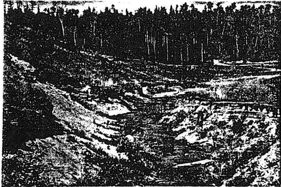
Figure 6. Extensive gulying in river terrace sands along the Athabasca River caused by surface runoff (west side of bridge on the Athabasca River - north of Fort McMurray).
