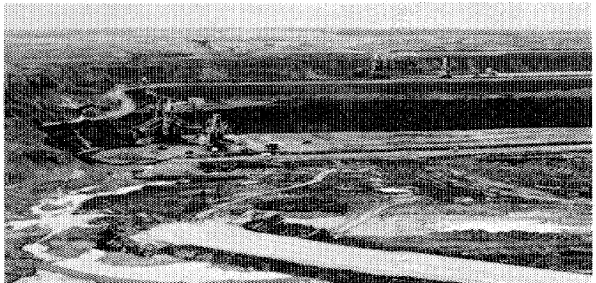
7 Bucketwheel excavators mining oil sands on the upper and lower benches in the Great Canadian Oil Sands pit.
