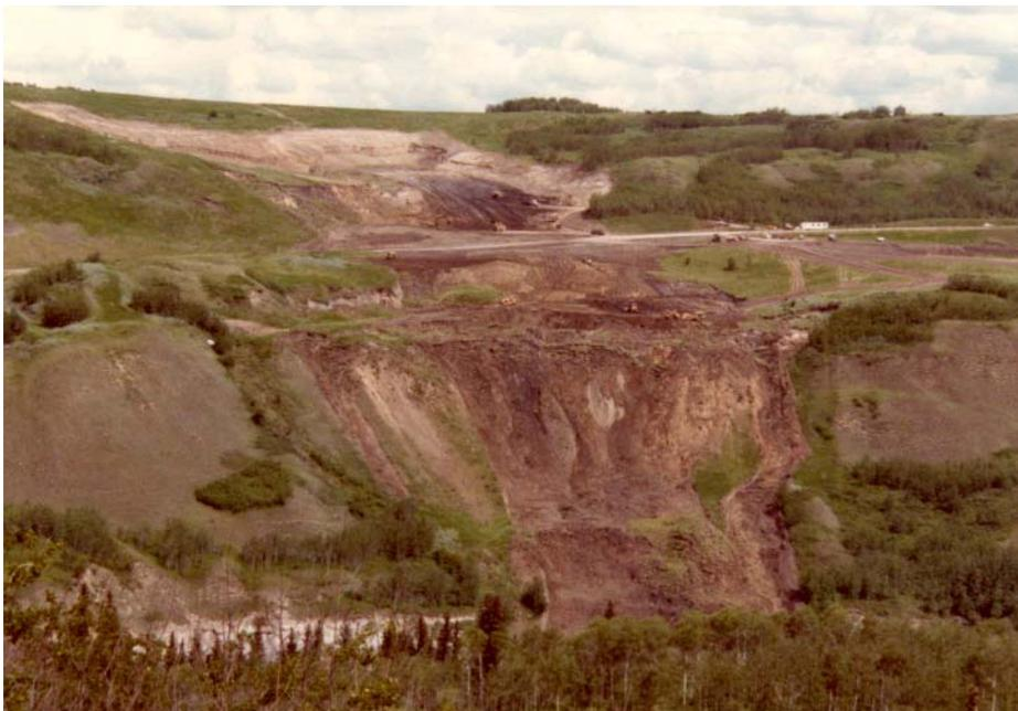
Figure 4. The 1984 earth flow (slide number 86) on the east Peace River hill (Highway 2) that partly dammed the Heart River (photo courtesy of Alberta Transportation 1985).
