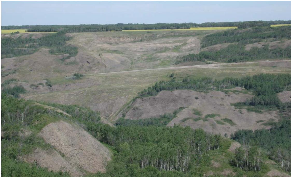
Figure 9. The 1984 earth flow, photographed in 2002 from across the Heart River. Highway 2 has been rebuilt across the landslide.
