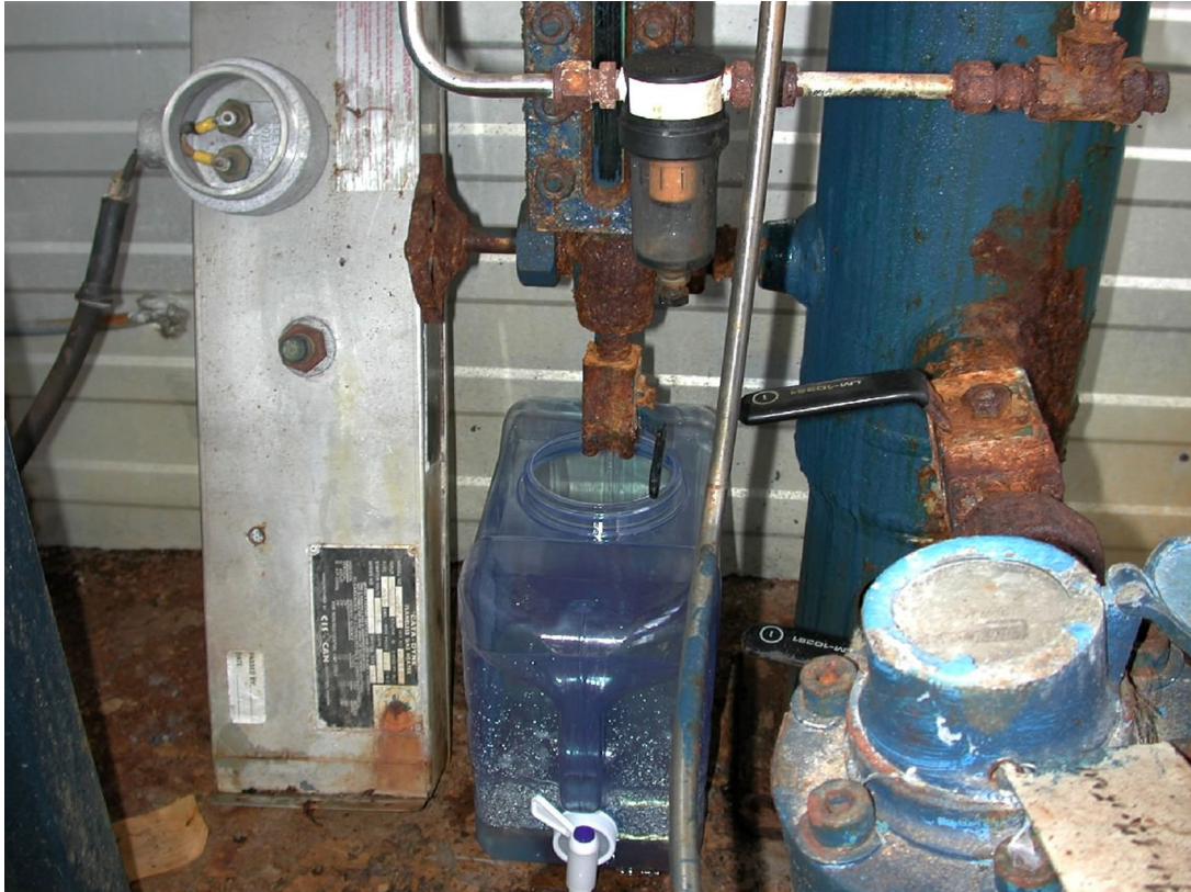
Formation water sampling set up
