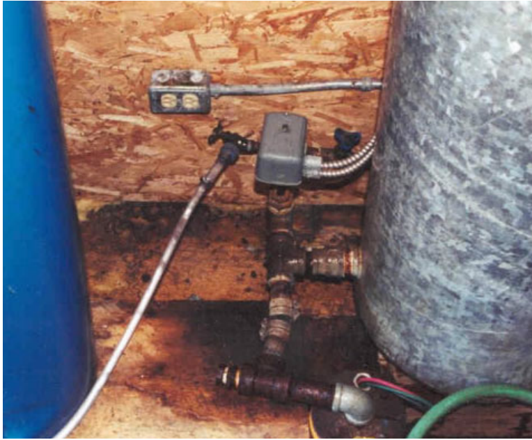
Figure 2. Connection of sample tubing to the water source.
