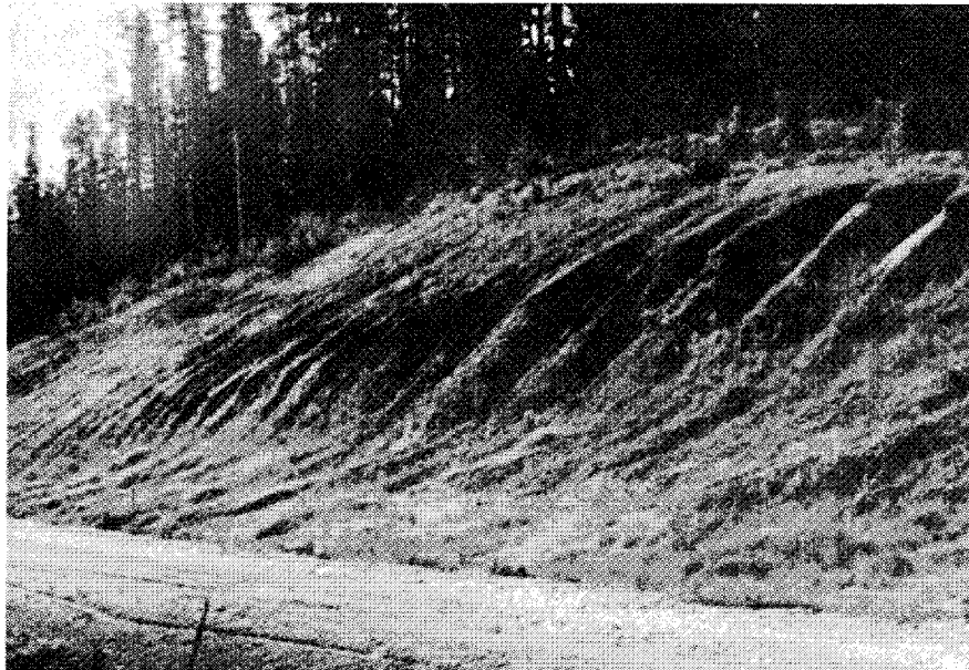
FIGURE 11. Extensive erosion of glaciolacustrine silts in the Swan Hills area to the south. 3 (Note how revegetation is occurring in spite of the steep slope.)
