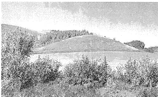
Plate 21. Areas easily erodible are kept in grass cover
