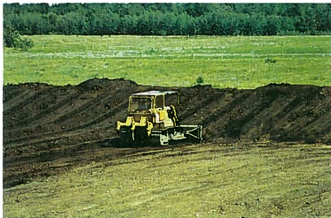
Plate 6. Pit south of Smoky Lake being stripped of soil. Soil should be replaced after extraction to bring site back into agricultural use.
